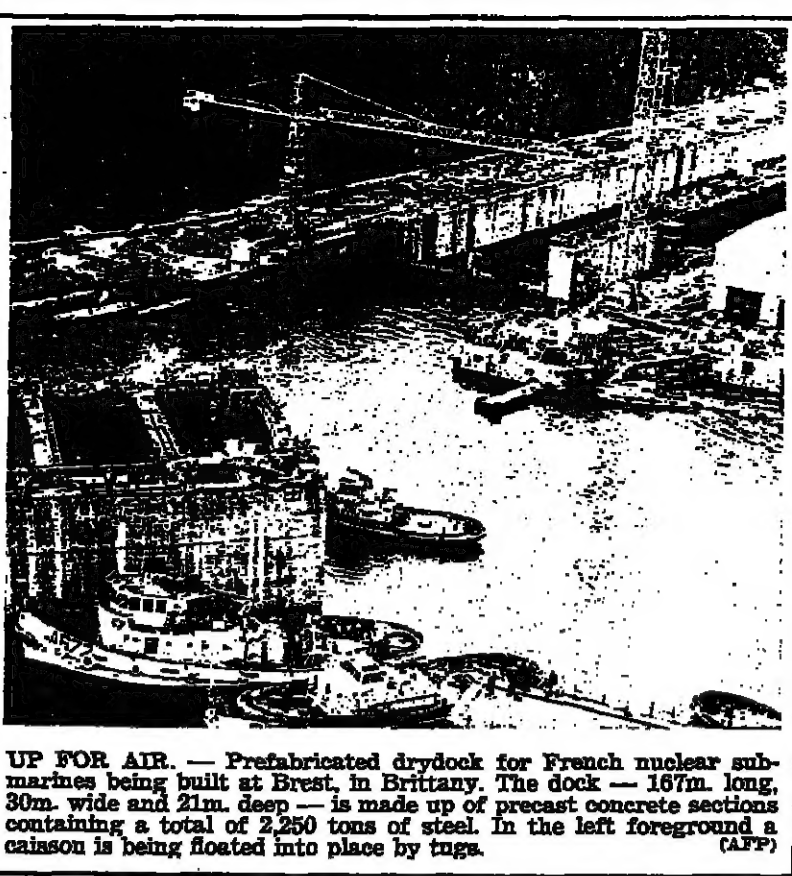
UP FOR AIR. — Prefabricated drydock for French nuclear submarines being built at Brest, Brittany. The dock — 167m long, 30m wide and 21m deep — is made up of precast concrete sections containing a total of 2,250 tons of steel. In the left foreground a caisson is being floated into place by tugs.
